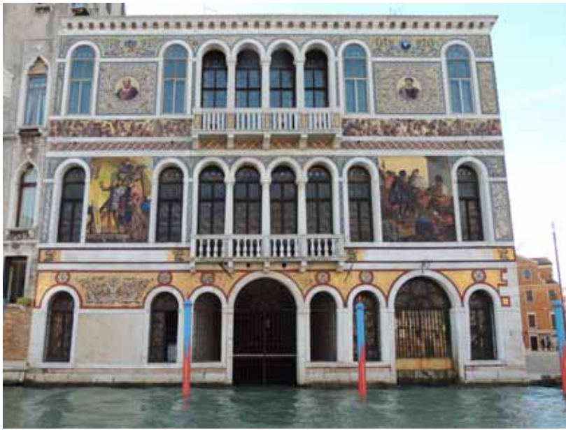
Palazzo Barbarigo, 16th century with 19th century facade
